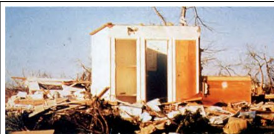
Interior rooms can be reinforced and retrofitted to be tornado “safe rooms”
