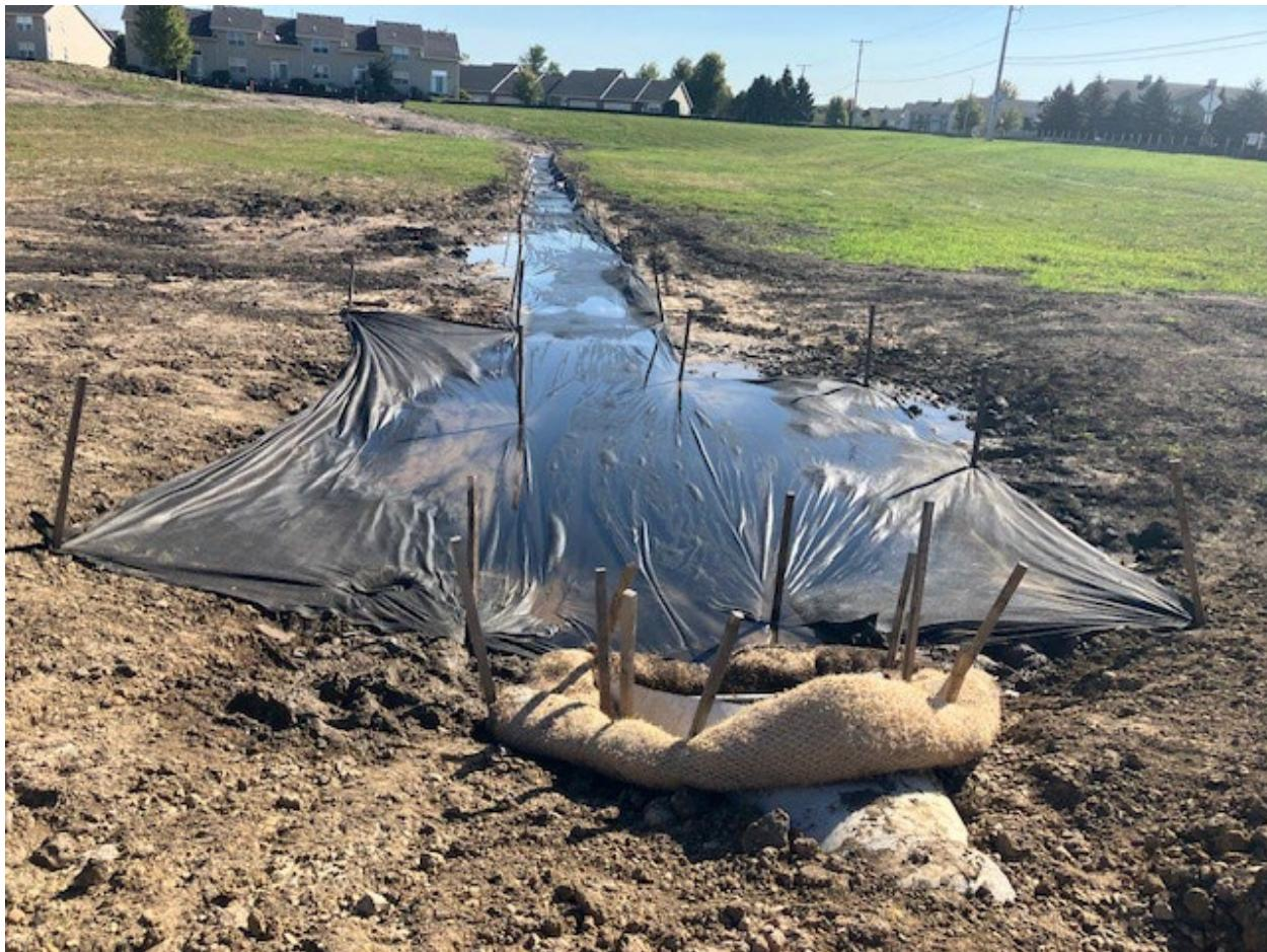
Improperly installed straw wattles. Sediment is passing below the wattle.
