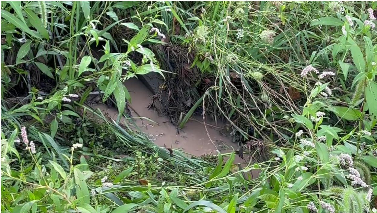
*Sediment rich water discharging from storm sewer into eastern ditch along IL Rt 23 near Mt. Hunger Rd.*
