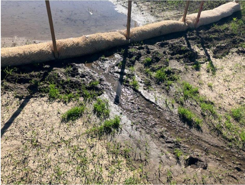
Incorrectly installed straw wattle. Runoff can pass directly under.
