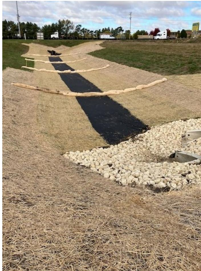
**Properly Installed and Overlapping Fiber Logs**
