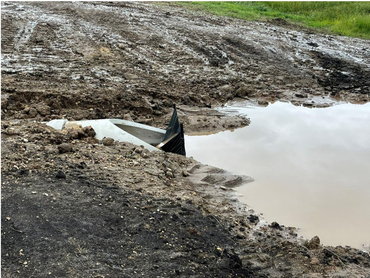
*Failing silt fence in eastern detention pond at Old Mill Park- North*
