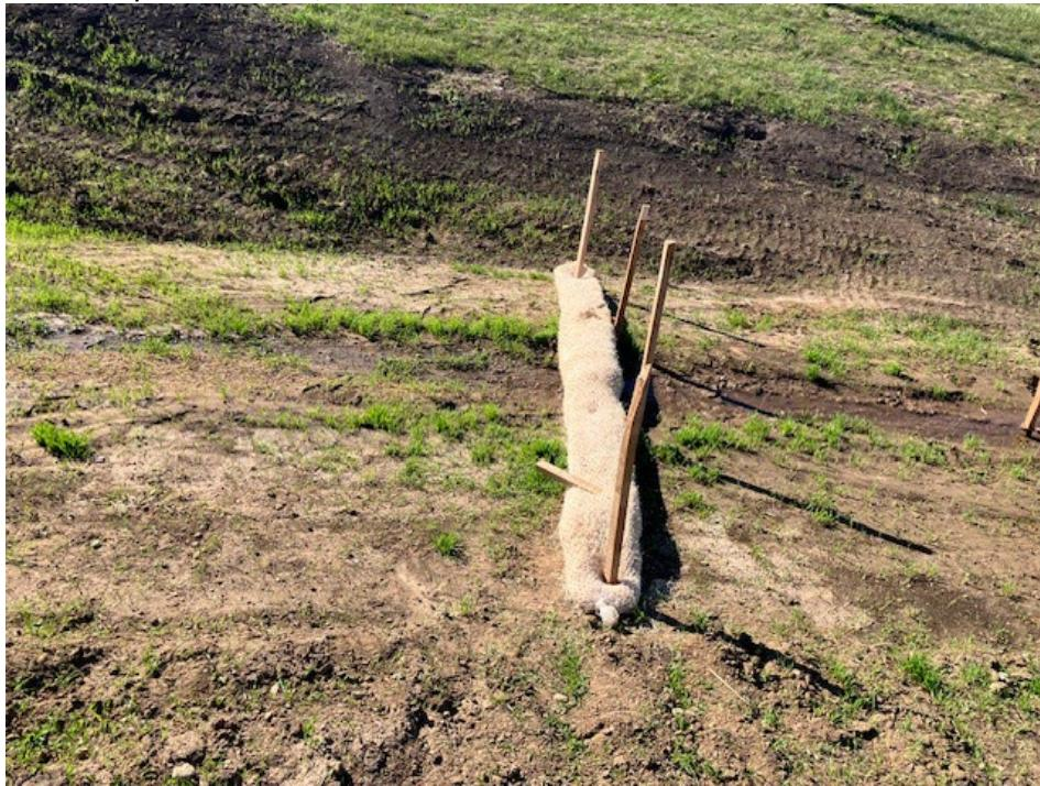
Incorrectly installed soil/erosion control. Note the bare earth downstream of the wattle.
